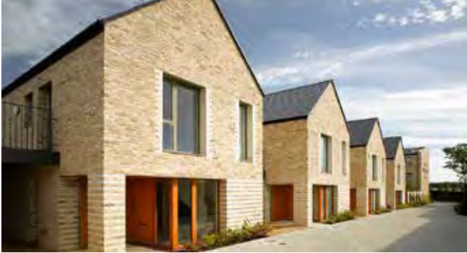
Figure 57; Example of dwellings fronting shared space
